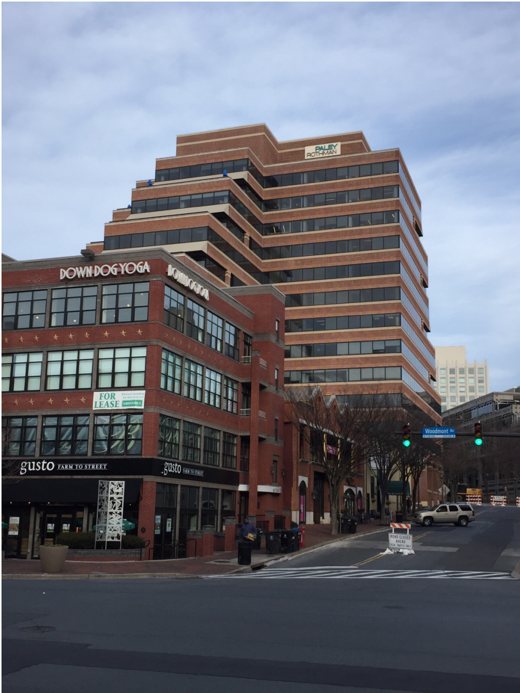
View of 4800 Hampden Lane from the corner of Woodmont Avenue and Elm Street.
